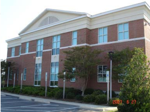
VIEW FROM JUNCTION OF OLD 64 AND NEW 64
